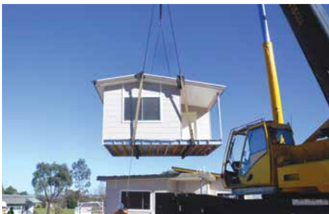
A home is craned into place in Coonamble
